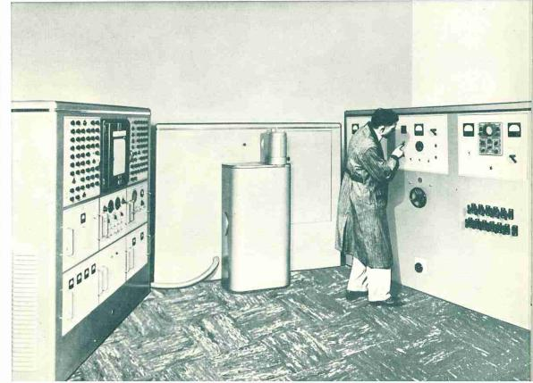
New, highly sensitive equipment, pioneered by Ladish Co., utilizing electronic dispatch and reception of ultra-sonic waves through water, automatically scans and records internal soundness of both steel billets and finished forgings.
