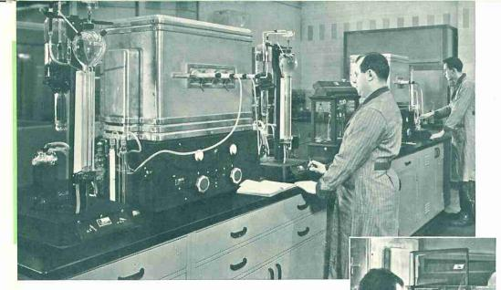
Since carbon is the most vital single element of steel, directly affecting strength, toughness, ductility and resistance to shock and abrasion, the Ladish Chemical Laboratory is equipped with advanced apparatus for accurate and rapid determination of the carbon content of steel.
