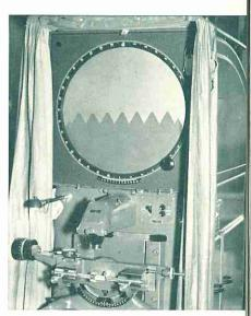
This Comparator provides an accurate means of comparing test pieces to known standards and thus contributes to safeguarding accuracy.
