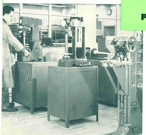
Hardness determination, accurately measuring the resistance of steel to penetration or surface deformation, forms an important corrollary of such desirable physical properties as strength, toughness and ductility and their proper balance. Various standard methods are used in the Ladish laboratory.
