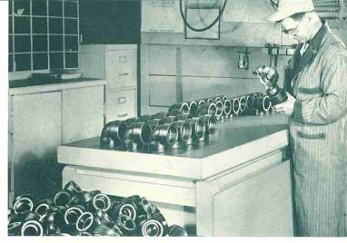
Evidence of thorough inspection methods is found in this gauging of the socket diameter of Forged Steel Socket Welding fittings. Final inspection completes a series of examinations which maintains Ladish standards of workmanship through all phases of production in full accordance with ASA Standard B 16.11.
