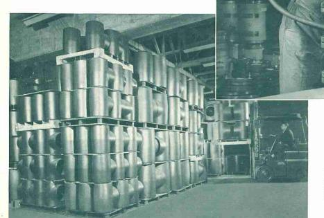
Bolting Ladish Flanges together into a compact shipping unit protects gasket surfaces and facilitates handling on the job.
